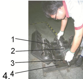
Picture 6-3: Installation of Bearing and Blade Rest 3
