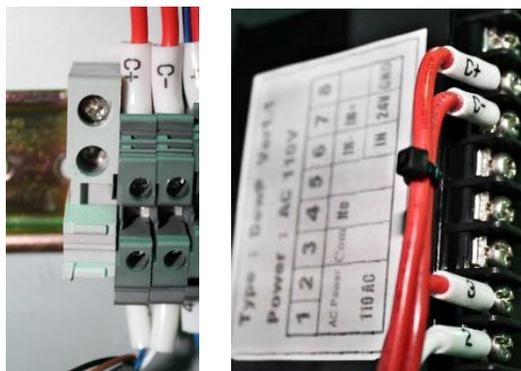
Picture 2-8: Connection of dew-point monitor
