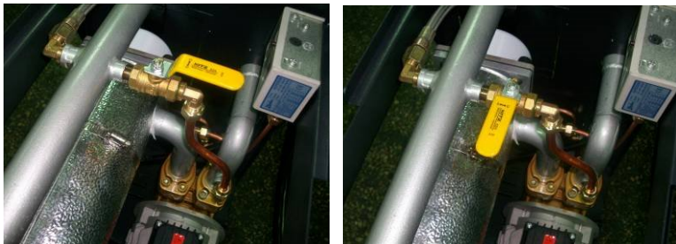
Picture 6-15: By-pass Globe Valve
