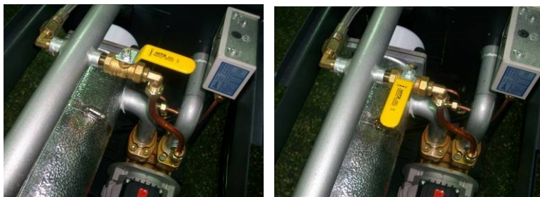
Picture 6-9: By-pass Globe Valve
