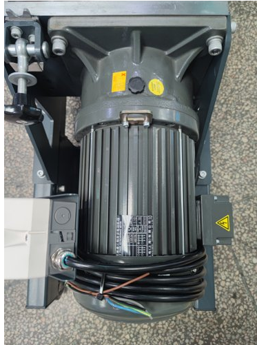
Picture 6-1: Motor Installation
