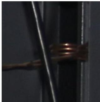
Picture 2-5: Capillary or Thermal Expansion Valve
