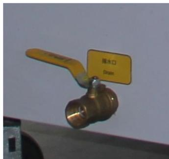
Picture 5-3: Water Drainage Port
