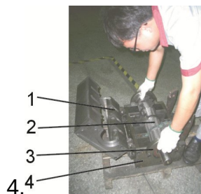
Picture 6-3: Installation of Bearing and Blade Rest 3
