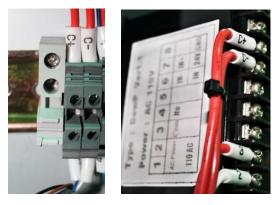
Picture 2-8: Connection of dew-point monitor
